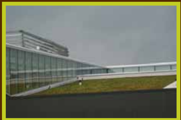
Part of the green roof. With the rain and heat of late summer, the plants on the roof flourished!
