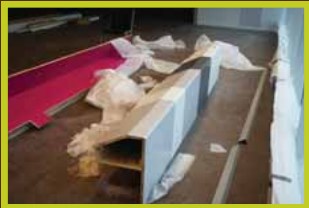
Special window benches for the children's area, ready to be installed.
